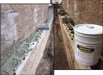
How are ProSpec Salt Barrier & Salt Barrier WB applied? ProSpec Salt Barrier & ProSpec Salt Barrier WB are applied using a low-pressure sprayer equipped with PVC, viton, or other compatible fittings and hoses. It should be applied evenly and sufficiently in order to wet the surface completely. Check out the video on the right to see the application process first hand.
